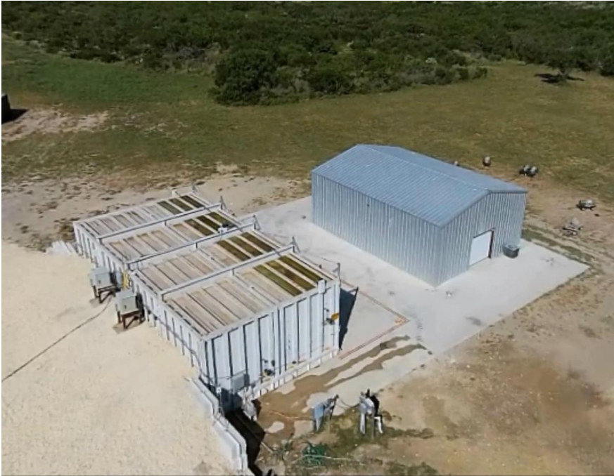
Full Scale PEMB TEST – Explosion Research Cooperative Box Canyon
